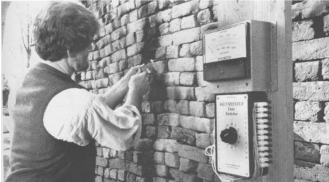
**Figure 1- A colonial interpreter installing a thermocouple into a kiln wall<sup>1</sup>**
