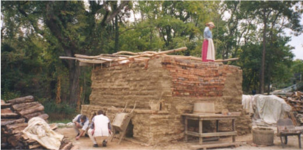
**Figure 12- Finishing the construction and daubing of the kiln**
